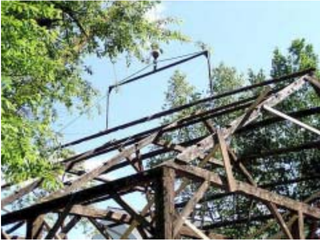
Icabod lifts the ridgepole from the frame.
