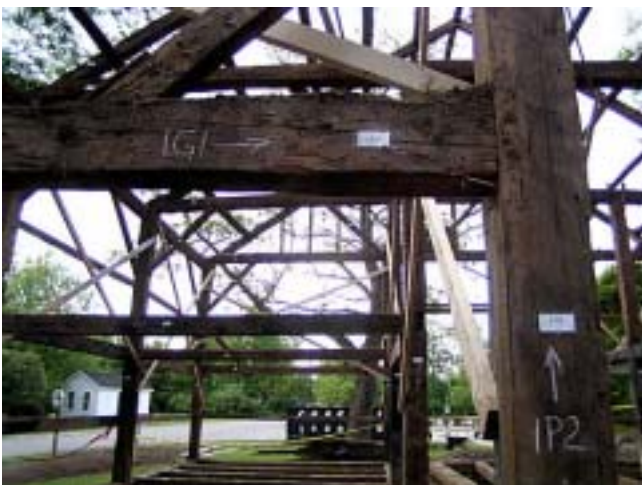
Each part of the frame was carefully marked so that reconstruction will be facilitated
