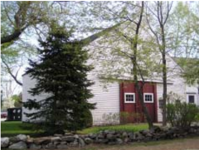
The barn before work began.
