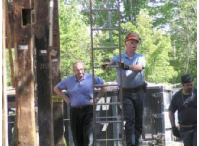
Chet Riley (on ladder) directed the barn's safe dismantling.
